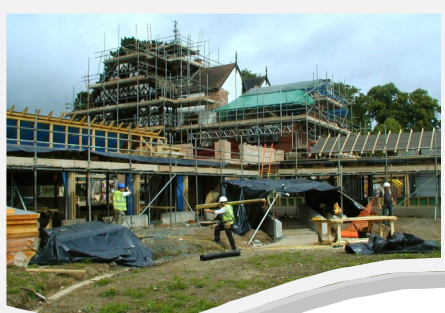
Work on the office wings at the rear of Grange Court
